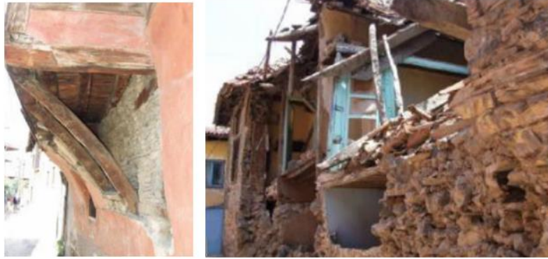
Figure 3. Bending and sagging in wooden material [25].
