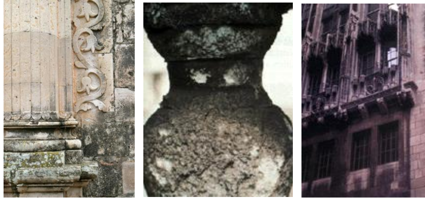
Figure 1. The effect of acid rain on stones [21-22]
