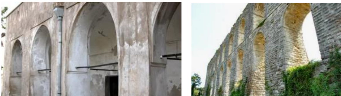
Figure 7. Deterioration in mortar and plaster materials [31].
